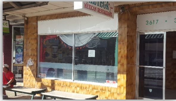
Figure 18 Fixed Window at 3617 Waialae Avenue
